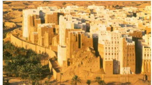
Yemen's Wadi Hadramawt village of Shibam is home to the world's first skyscrapers. A cluster of 500 mudbrick, stone, and wood residences, some eight stories high, Shibam's tall structures pre-date the Industrial Age by many centuries, earning the moniker bestowed upon them by the famed traveler Freya Stark as the "The Manhattan of the Desert."
