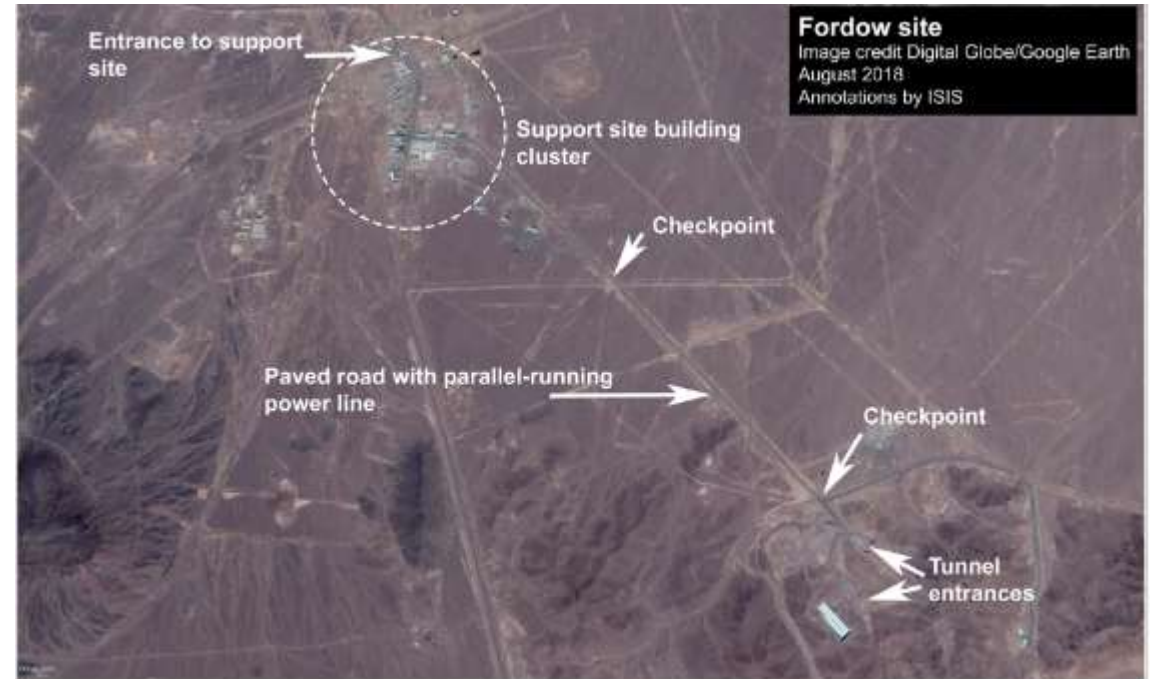
Figure 2. Overview of the Fordow facility, which includes the underground tunnel complex and the support complex.
