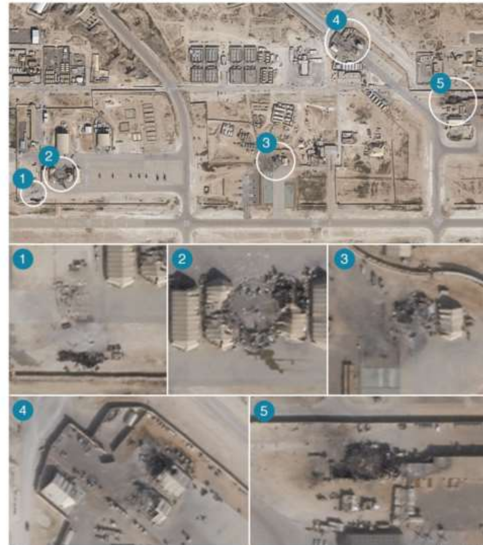
Damage and destroyed structures at Al Asad Air Base
